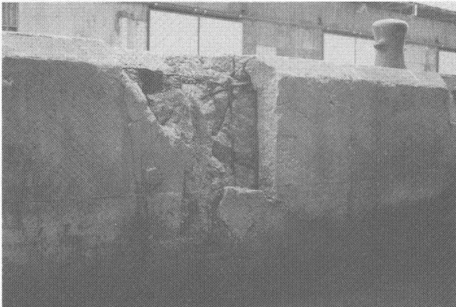
Figure 1-7. Deterioration of sheet pile bulkhead in a marine environment. (a) Corrosion of steel sheet piles in splash/tidal zones. (b) damaged concrete cope wall. (c) concrete erosion by moving sediments.
