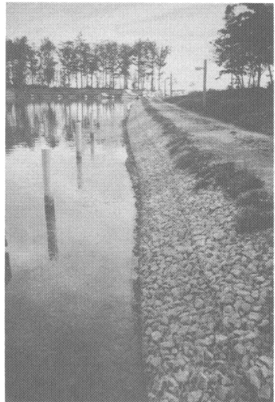
Figure 6-54. Typical slope armoring. 1—Rip-rap, 2—filter cloth, 3—interlocking blades, 4—concrete paving.
